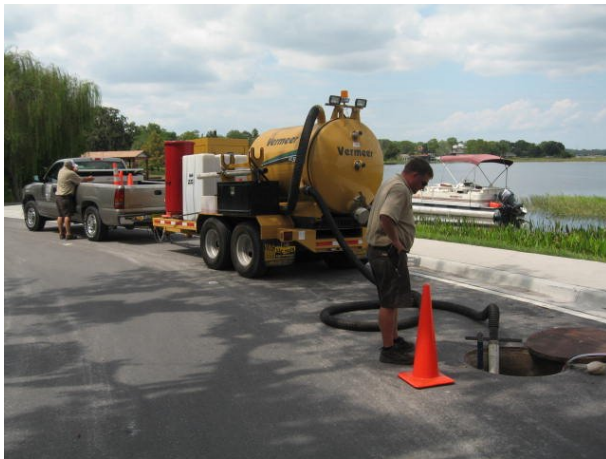
a. Manhole Cover Removed to Access Unit
