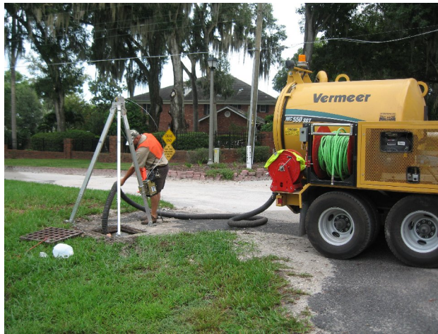
a. Inlet Cover Removed; Worker Enters Using Harness
