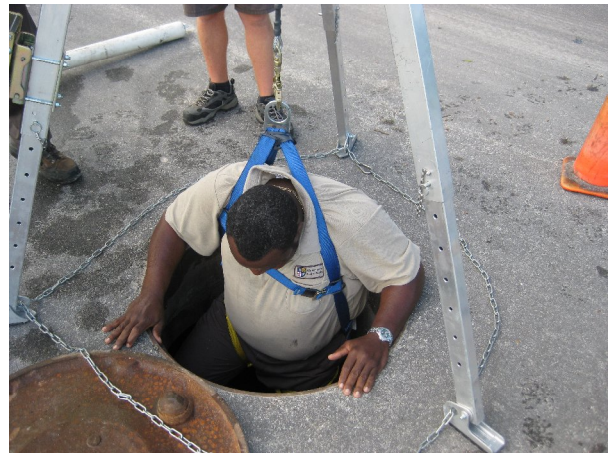
b. Worker Lowered by Harness into Unit
