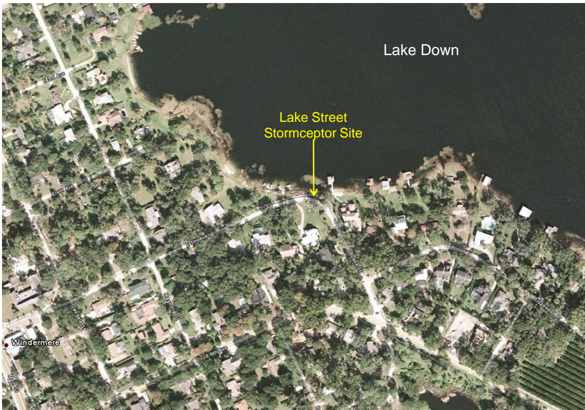
Figure 1-7. Overview of the Lake Street Stormceptor Site.
