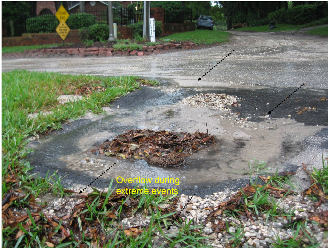
Figure 2-2. Inlet Structure for the Pine Street Site.
