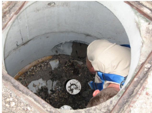
b. Pipe Removed to Access Sump Area
