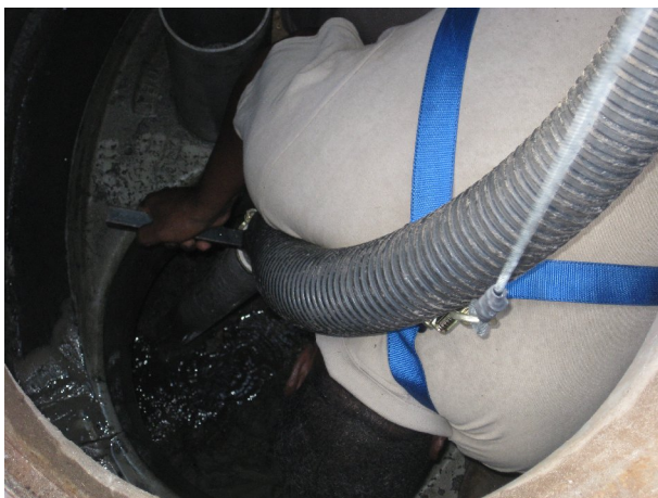
c. Metal Grate Cover is Raised to Access Sump Area
