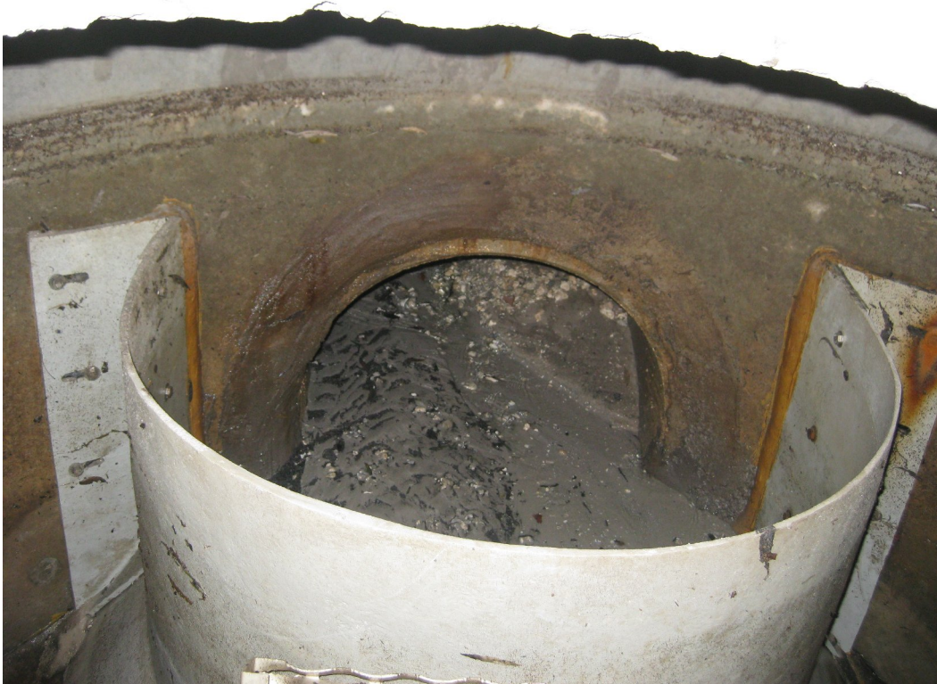
Figure 1-13. Diversion Weir for the Lake Street Stormceptor Unit.
