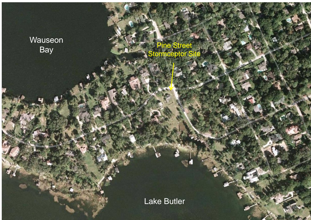
Figure 1-4. Overview of the Pine Street Stormceptor Site.
