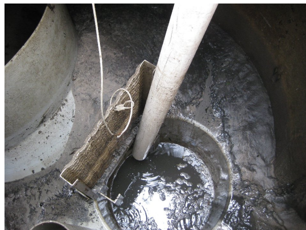
d. Suction Hose Inserted into Sump
